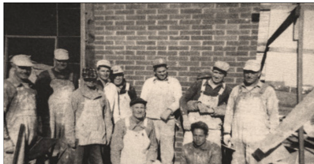
Builders of the first meetinghouse in Moses Lake for The Church of Jesus Christ of Latter-day Saints (1950)
